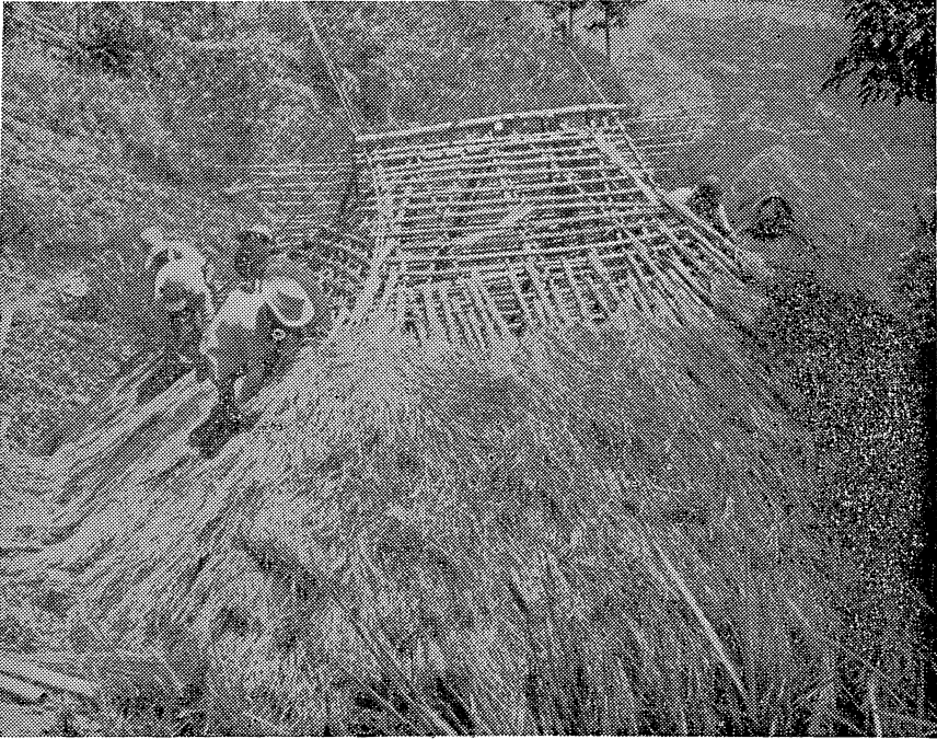
Plate 1. The roof of an apa dwelling under construction.
