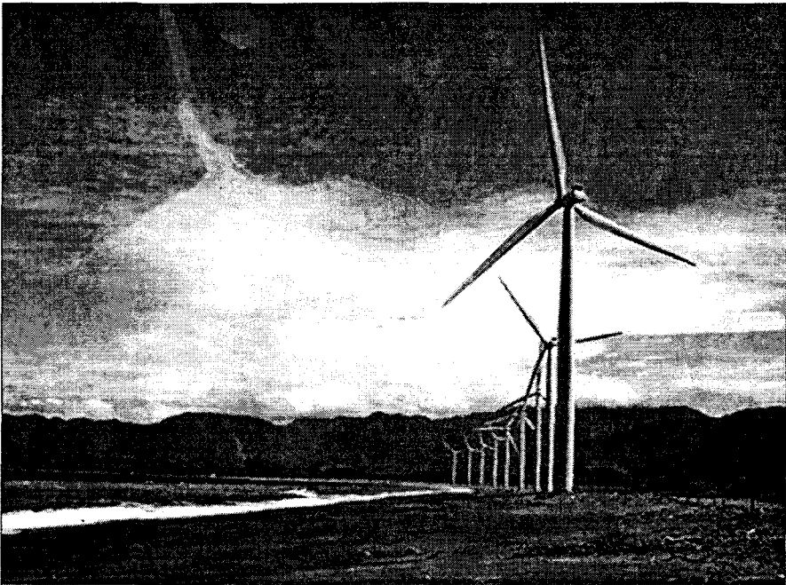
FIGURE 14. The wind farm in Bangui Bay, Ilocos Norte. Photograph by Tonie Santos.
